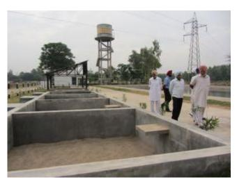
Figure 4-2 Sludge drying beds, with the third oxidation pond in the background.
