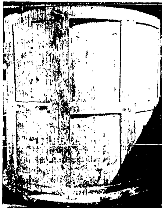
Ferrocement water tank - capacity 20000 litre, constructed using SERC segmental technique.
