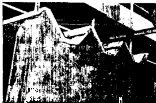
Ferrocement trough shaped precast roofing units for span upto 5.0 m - cast using SERC mechanised process.
