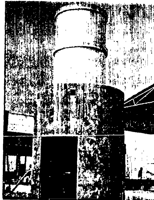
Ferrocement water tank - capacity 2500 litre used as overhead tank in a pipe factory in NOIDA. Produced with SERC semi- mechanised process.
