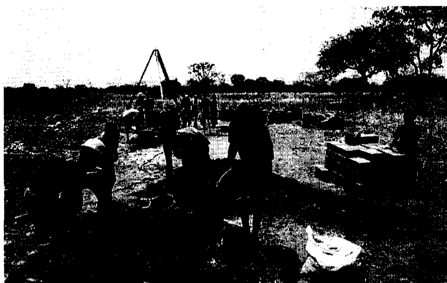
Bugya Tinkura village near Walwale, Ghana. A team of villagers construct a hand-dug well. The men in the foreground are mixing cement and aggregate, which has been broken by hand, to make concrete for caisson rings to line the well, seen in background.
