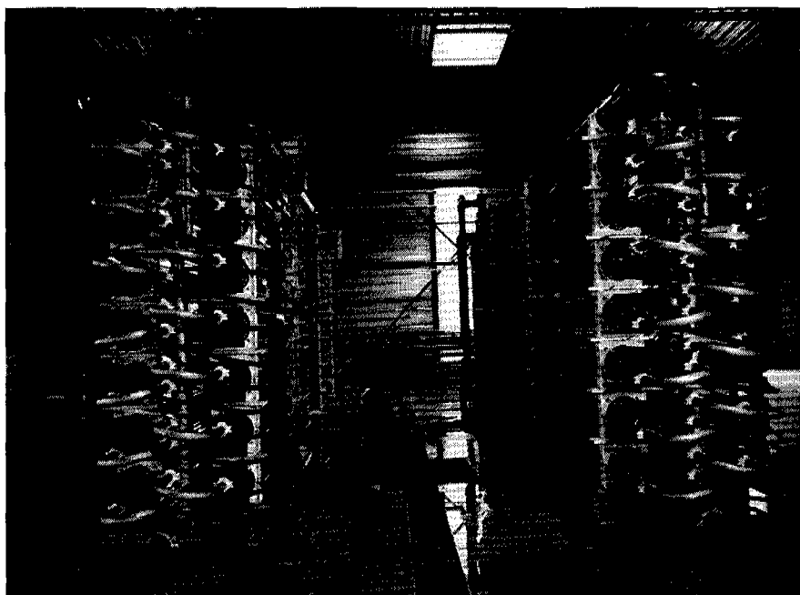
Figure 2. Nanofiltration at Méry-sur-Oise.
