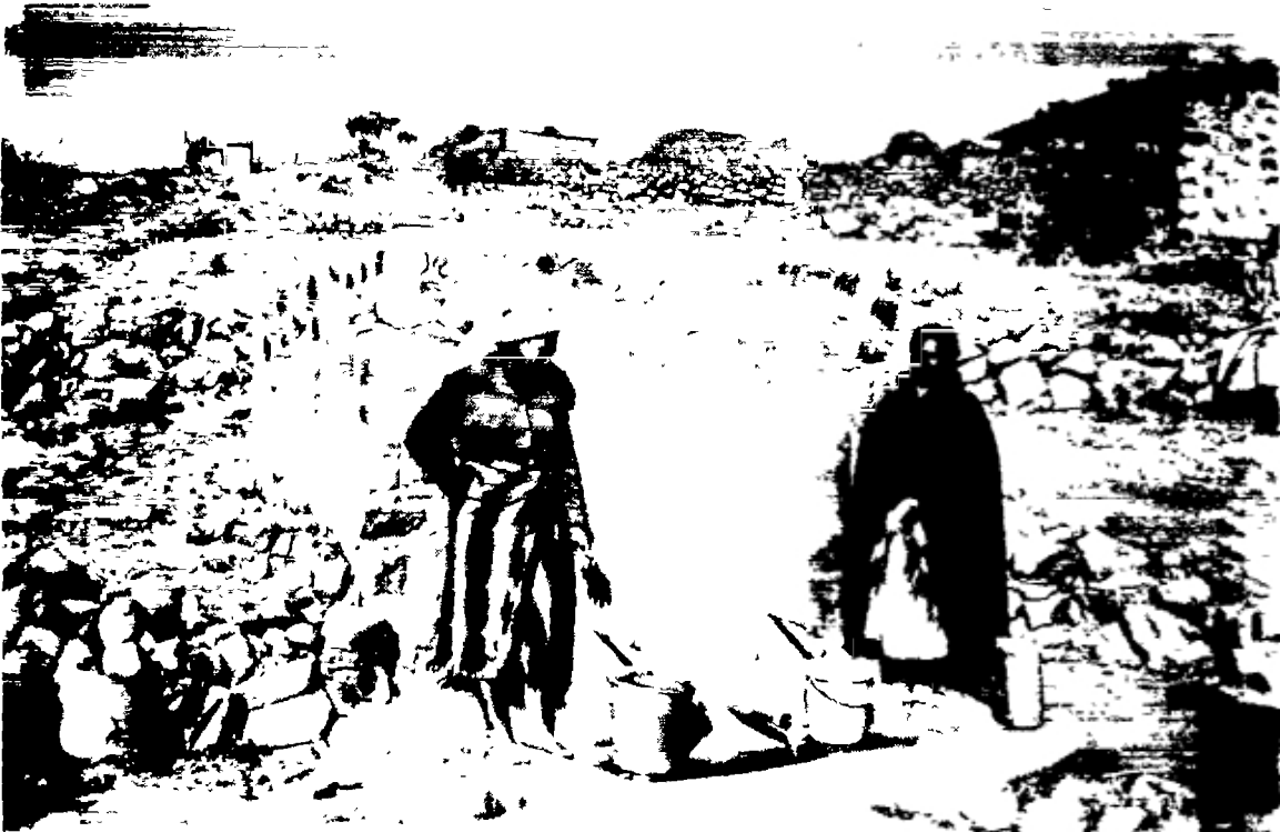
Collecting water from storage tank at Motsolwane
