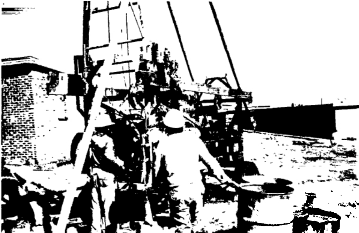
Local drillers building water well at Ha Sekepe
