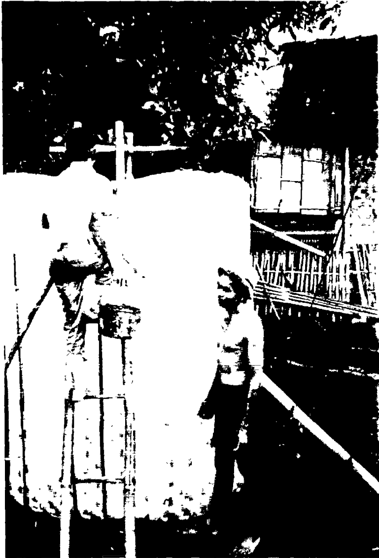
Building a water storage tank using CARE project skills and self-financing.
