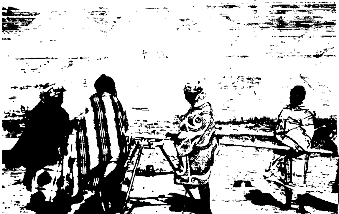
Women cutting pipe for water system at Linakeng
