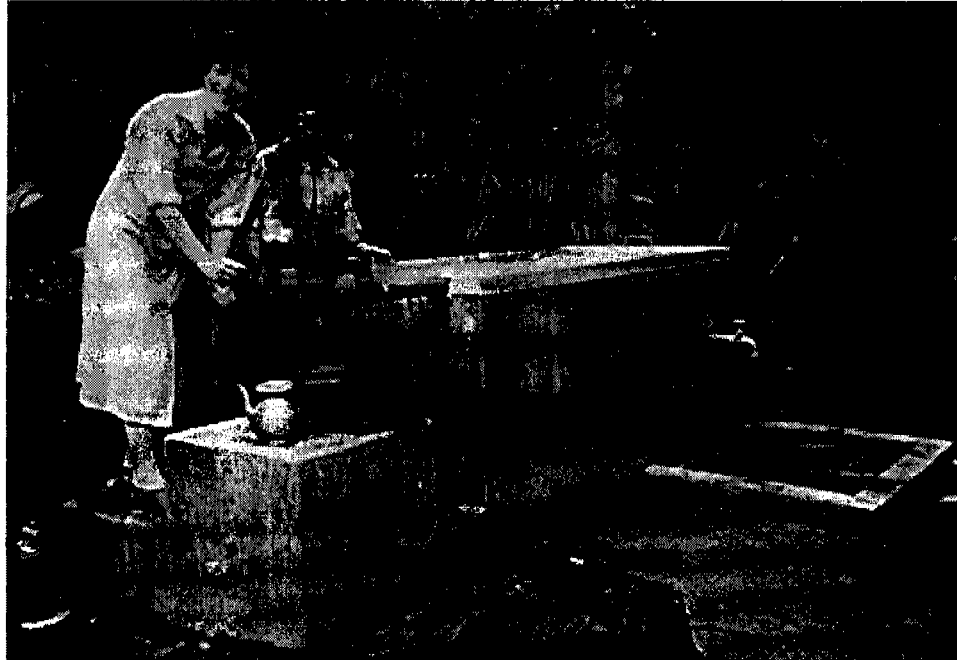
Figure 1 Iron-Arsenic Removal Unit attached with Handpump
