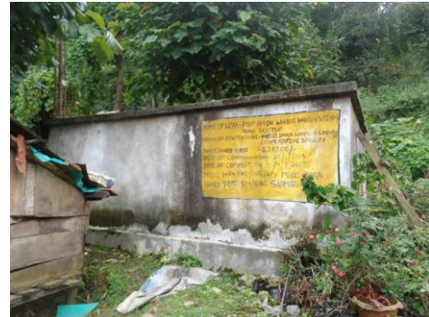
Tank constructed under Roof Rainwater Harvesting Programme- also used as storage tank for drinking water
