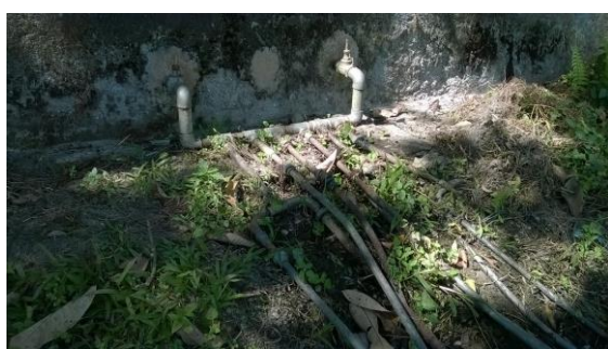
Photos: Distribution lines from distribution tanks
