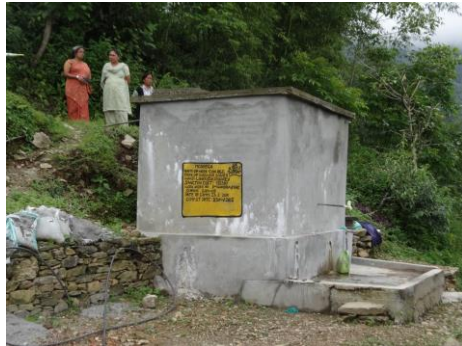
Tank constructed under Roof Rainwater Harvesting Programme- also used as storage tank for drinking water
