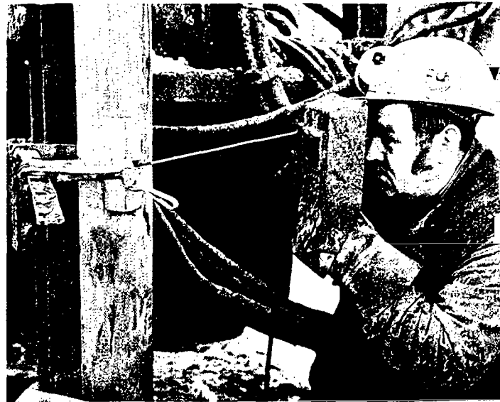
Fig. 53. Welding of casing tubes
