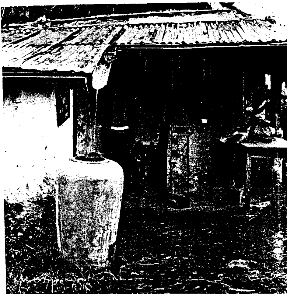
Fig. 2.1 Simple Roof Catchment
