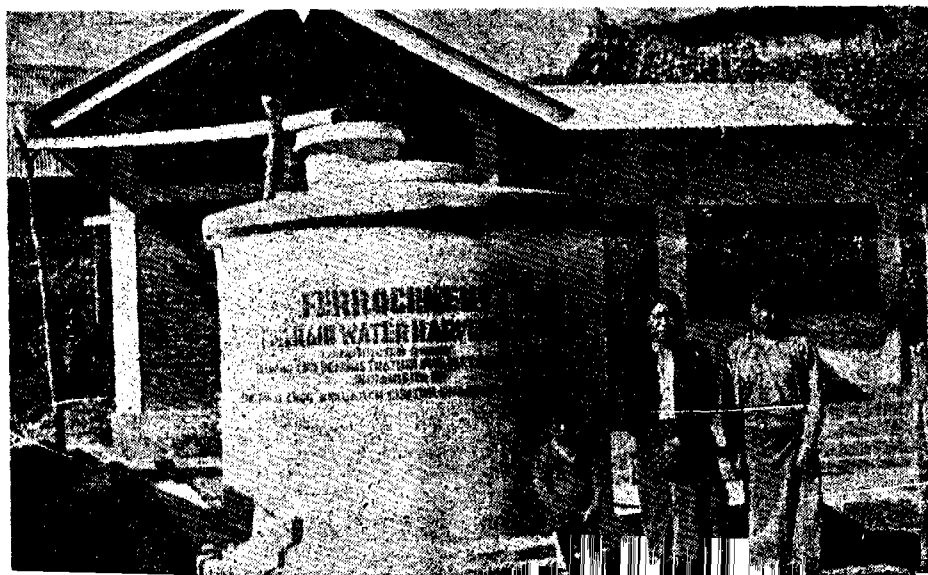
Fig. 8. A ferrocement tank for rain water harvesting installed by SERC, Ghaziabad.
