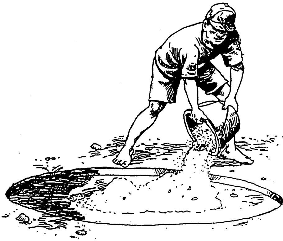
H6: Fill the hole with the concrete
