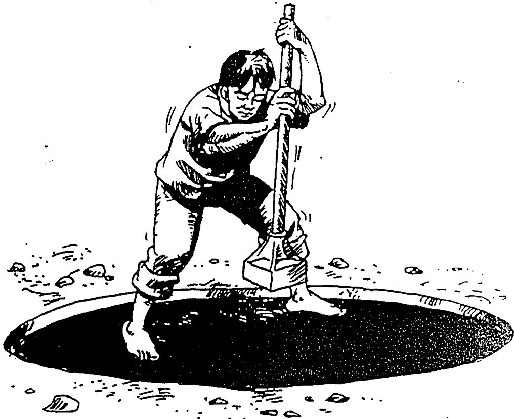
H5: Compact the sand filled to have a layer of 10 CMS.
