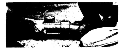
Insert the pipe into the socket, turning gently Wipe off excess solvent cement
