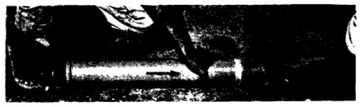
— Join the cylinder to the bottom of the first length of rising pipe Push the cylinder firmly in as far as possible, but do not hammer it in Leave at least 10 min. to dry before handling.
