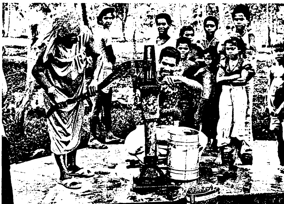
PLATE 6: The pump at Guaco after replacement parts had been installed.
