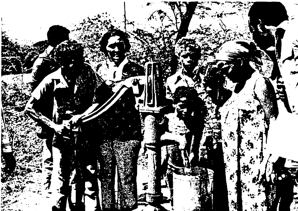
PLATE 4: New installation at El Medio.
