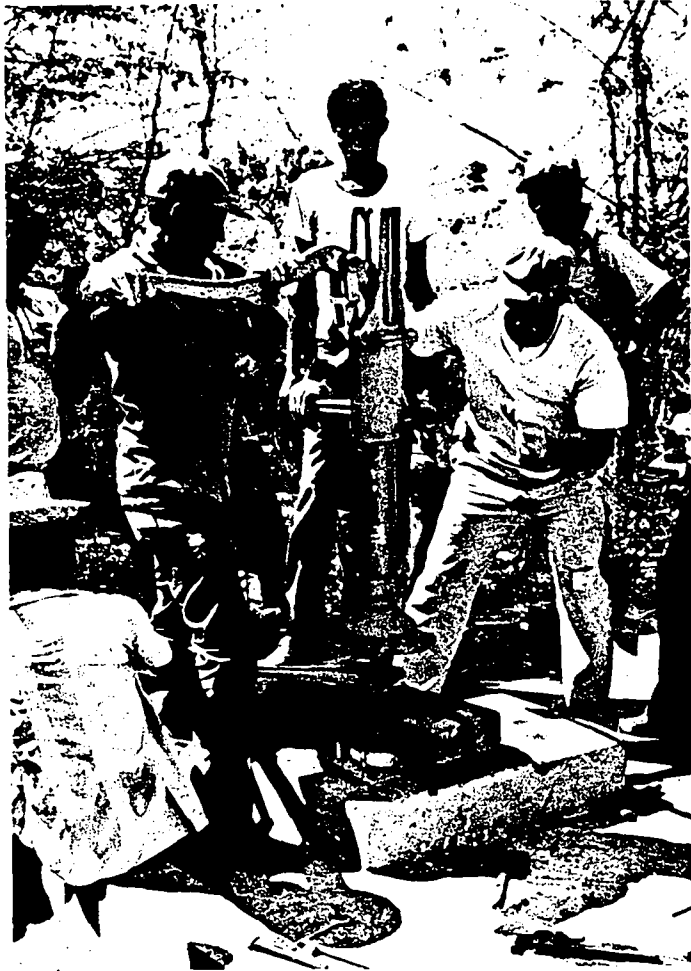
PLATE 3: Pump being installed at El Barro.
