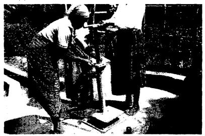
xvi) Connect the sleeve bearing onto the pump stand by hand and then tighten it by F-key.
