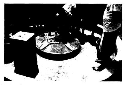
ii) Put the base plate onto the archor bolts on top of the gasket.
