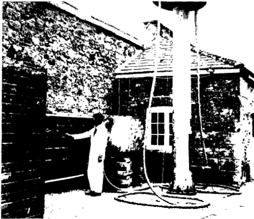
Figure 5.2 Solar Pump Test Facility – Office and base of 18m high mast showing delivery tank
