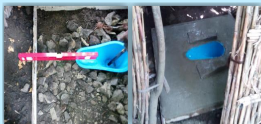
Figure 1: SATO skirting on wooden platform
