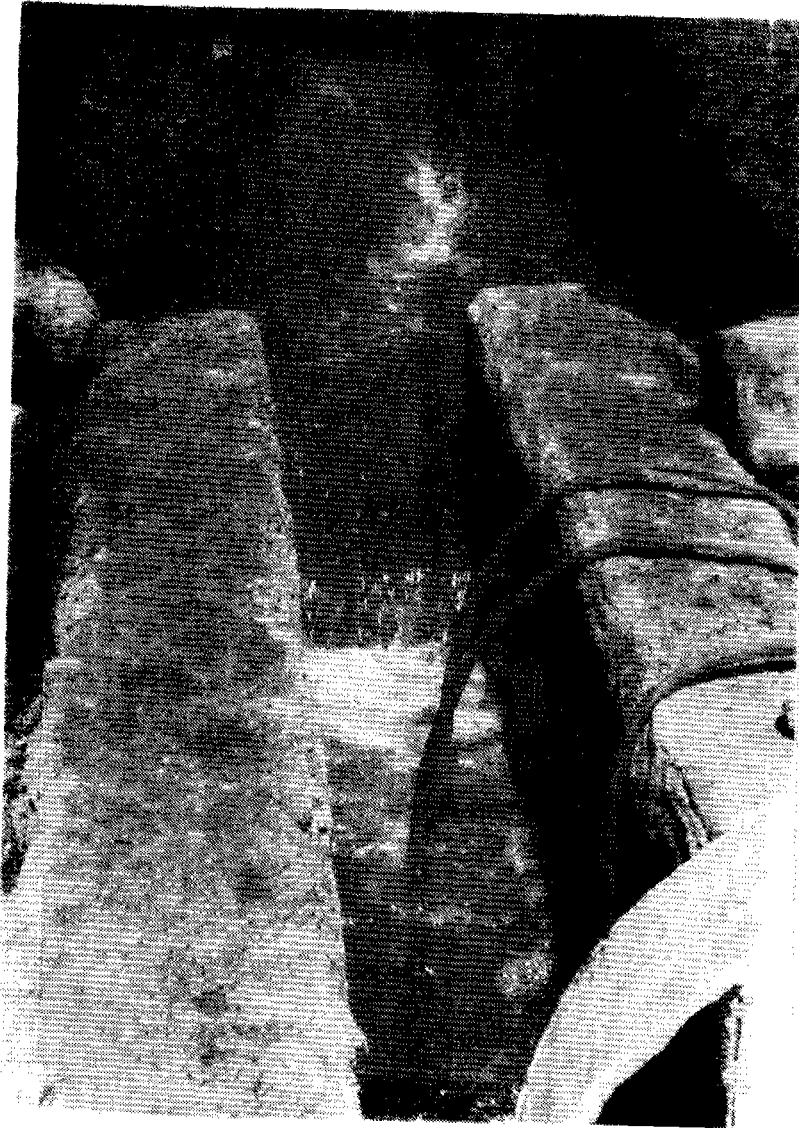
Figure 4.14 Drop and turbulent flow in the inlet channel.
