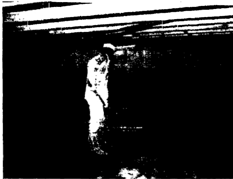
Figure 2.2-3: The scraping operation during cleaning of slow sand filters
