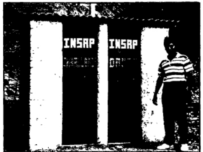
These improved latrines were constructed with community participation and are kept clean by community volunteers in a project near Lima, Peru. (EHP/Robert Varley)
