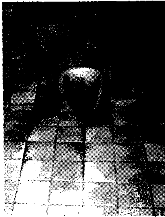
Inside of a tiled pour-flush toilet
