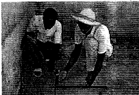
Setting out of latrines
