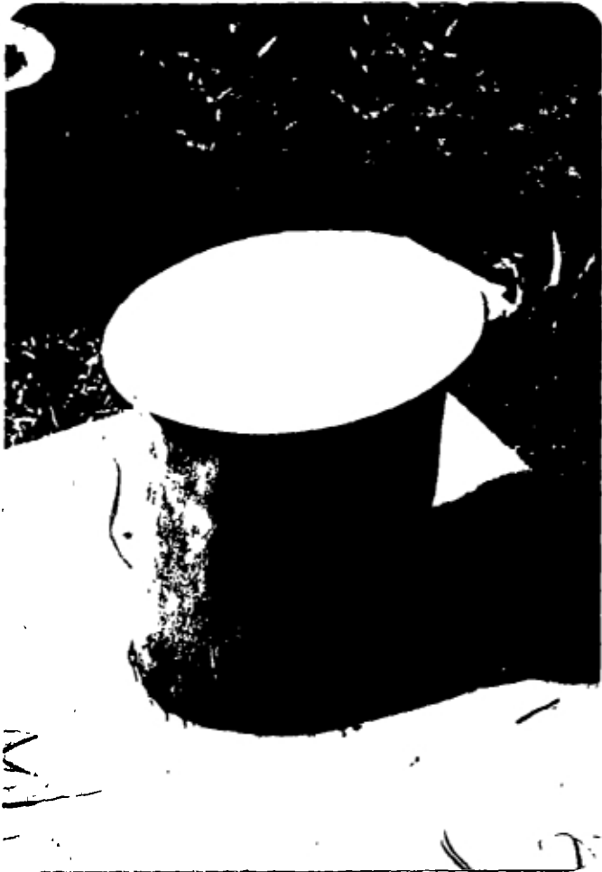
Latrine riser used with pour-flush polythene bowl (Photo 15)
