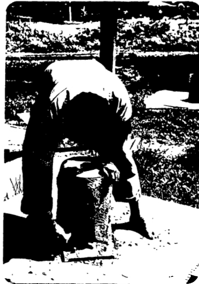
Precasting of latrine riser by plastering (Photo 6)
