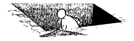
• Use a bucket and rope to remove earth from the pit. Heap the earth two metres or more away from the pit.
