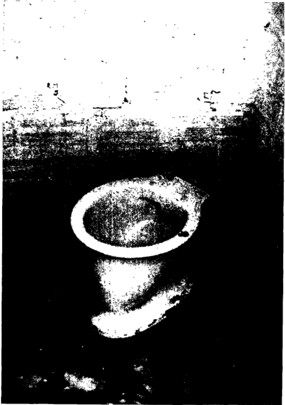
Figure 4. Ceramic pedestal latrine unit for use either in pour-flush mode (as above) or, when connected to a small cistern, in cistern-flush mode (Brazil).
