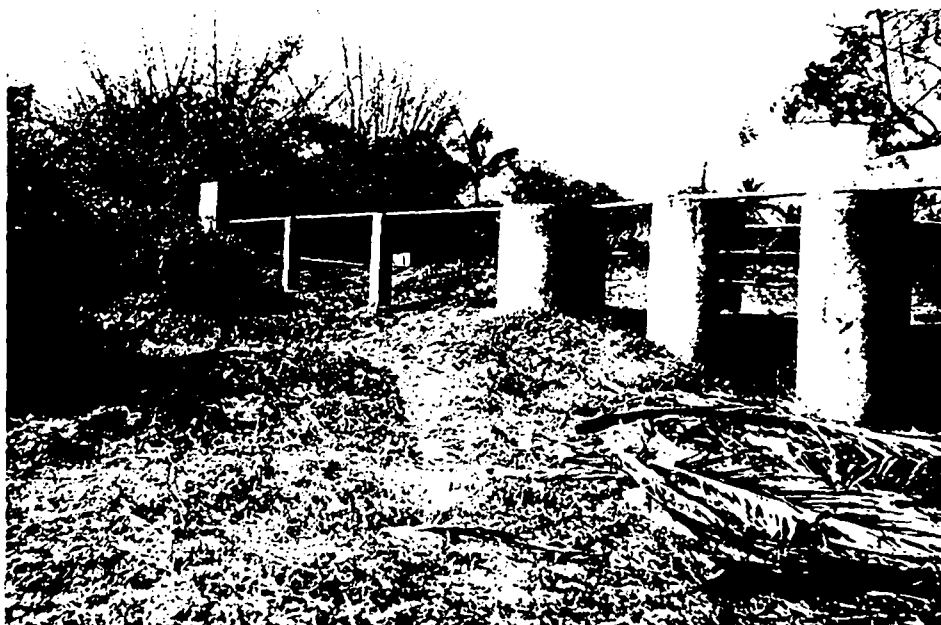
Fig. 1. Stabilization ponds made of cement cisterns operated at 1.22 m (A), 1.83 m (B), and 2.44 m (C) depths.
