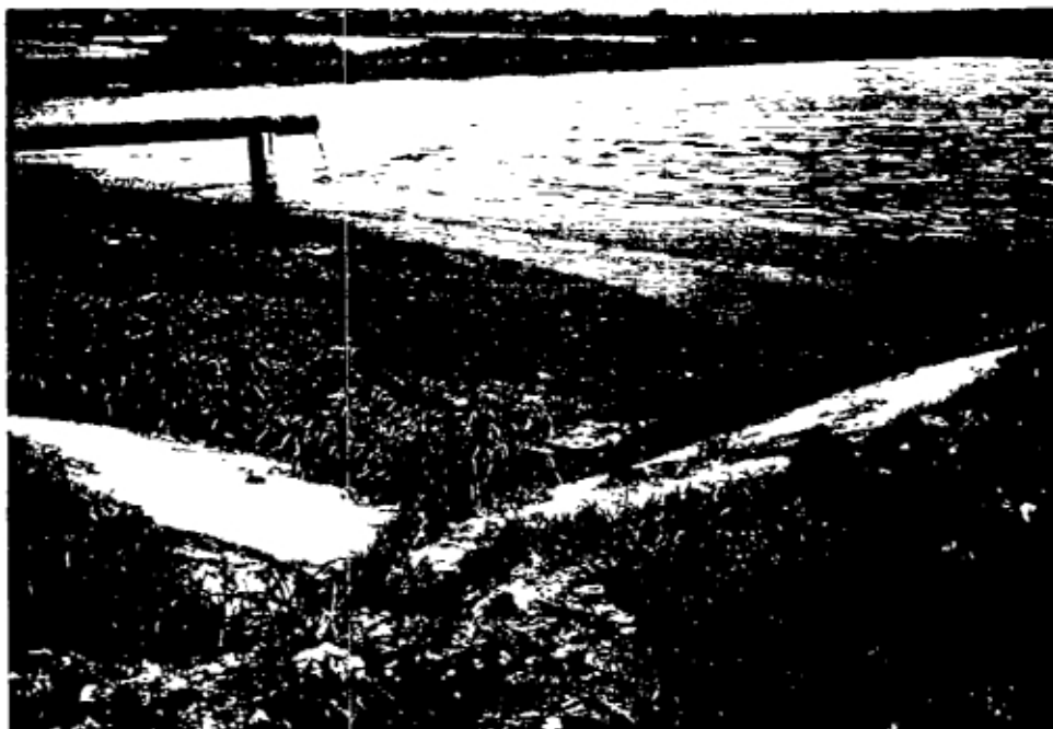
Figure 10. A view of the Vingunguti anaerobic ponds showing the inlet pipe and scum accumulation.
