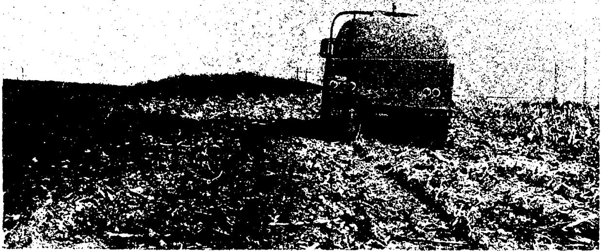
Figure 10-8. Tank truck with side spray nozzle for liquid sludge surface application (17).
