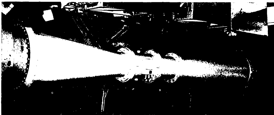
FIG 2 ELECTROMAGNETIC FLOWMETER INSTALLED BETWEEN PIPE TAPER PIECES
