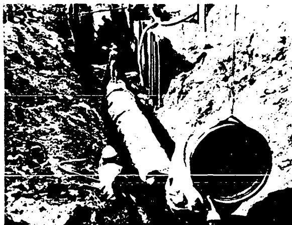
Figure 6. Construction of the Caroni-Arena Transmission Pipeline System. The 85-km route of the arterial system traverses developed areas and intersects numerous roads, underground utilities, drainageways, and small streams. The photo shows crews installing pipe at a drainage undercrossing.
