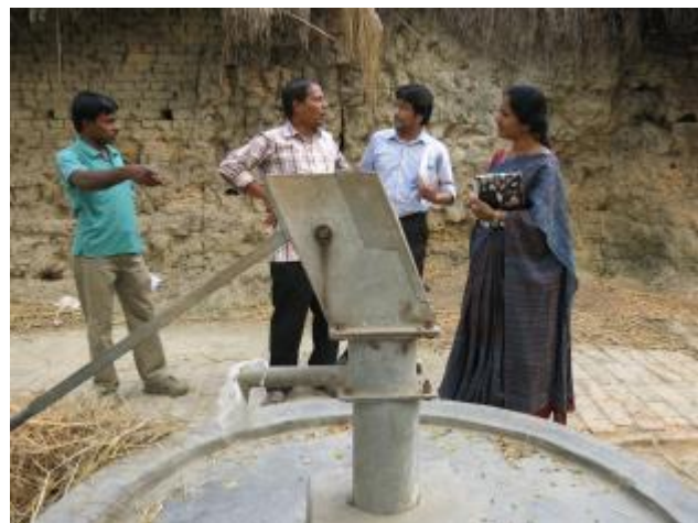
Photo 4: Users in Durganagar Kanchantala explaining problems with the unrepaired handpump
