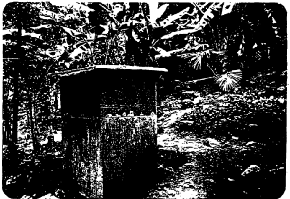
Seelatenna - A completed latrine.
