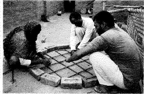
▲ Najafgarh workers prepare steel rods for strengthening a cement latrine platform.
