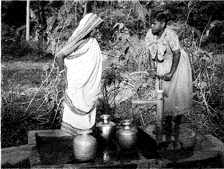
The Tara is the optimum pump for alluvial areas (Bihar).
