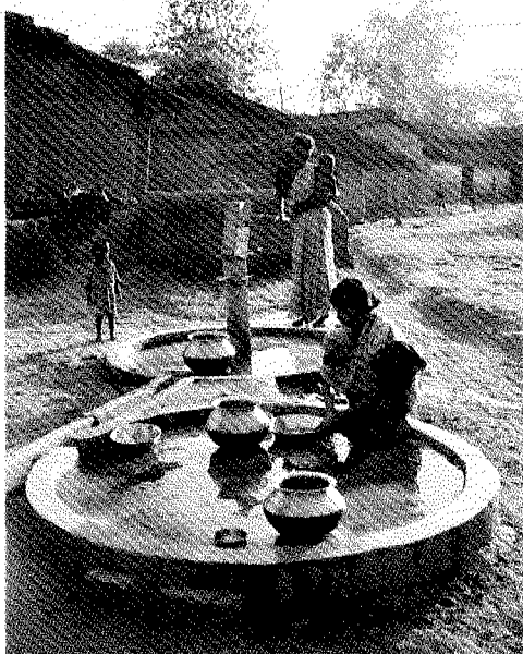
A separate washing platform helps to keep the area around the pump clean.
