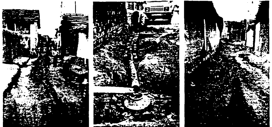
'Before' and 'after' soakpits
