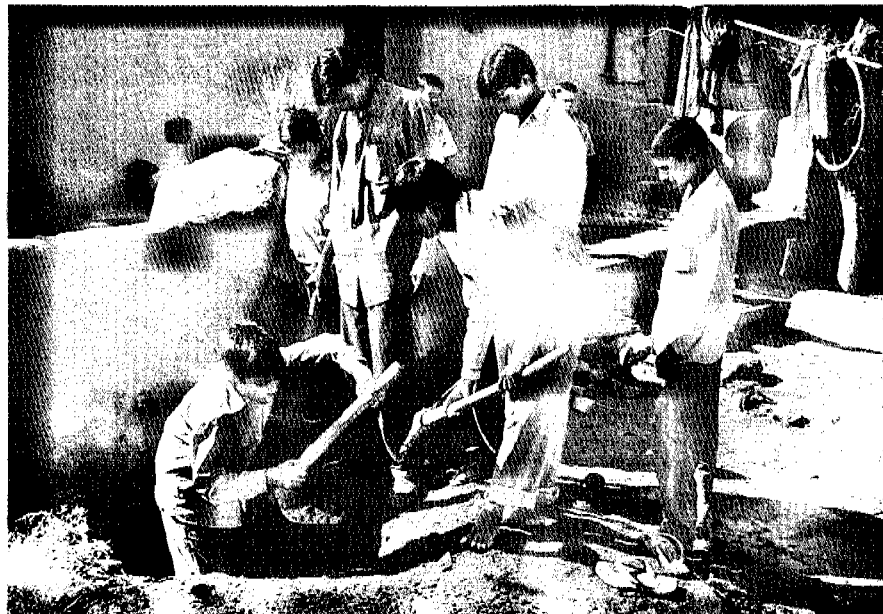
School students dig a shauch khadda (trench pit toilet) at Dahegaon village
