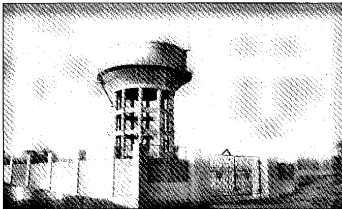
Elevated Supply Reservoir
