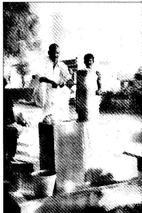
Repairing of Taps by Village Caretaker
