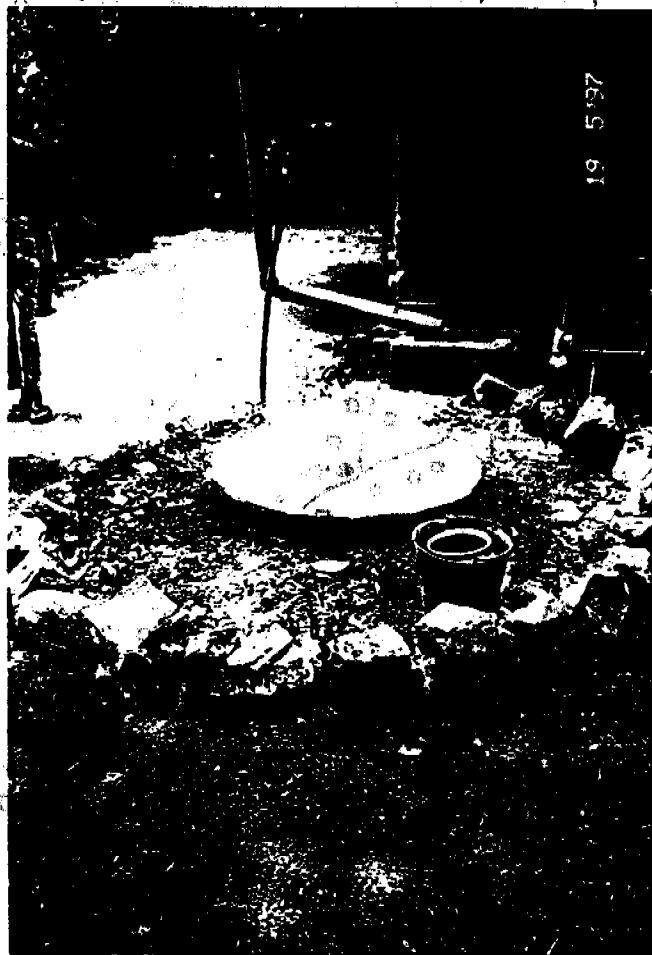
Surface opening of a under ground brick-dome tank
