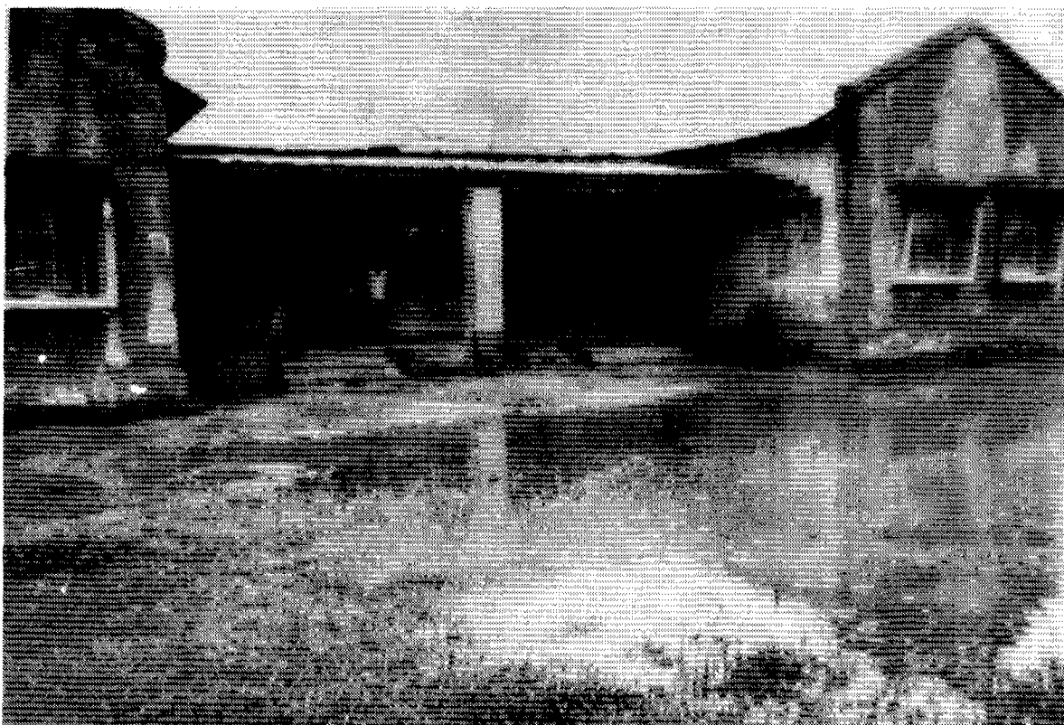
Stagnated rain water that accumulated because of lack of drainage is seen in front of this primary School at ward no. 19.
