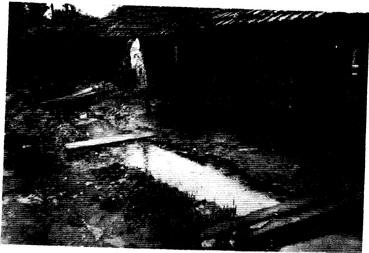
Poor drainage in front of the houses in Ghogapul.
