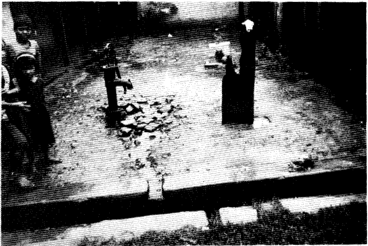
A makeshift 'canal' allows the tubewell's waste water to go down the drain which has no final outlet.
