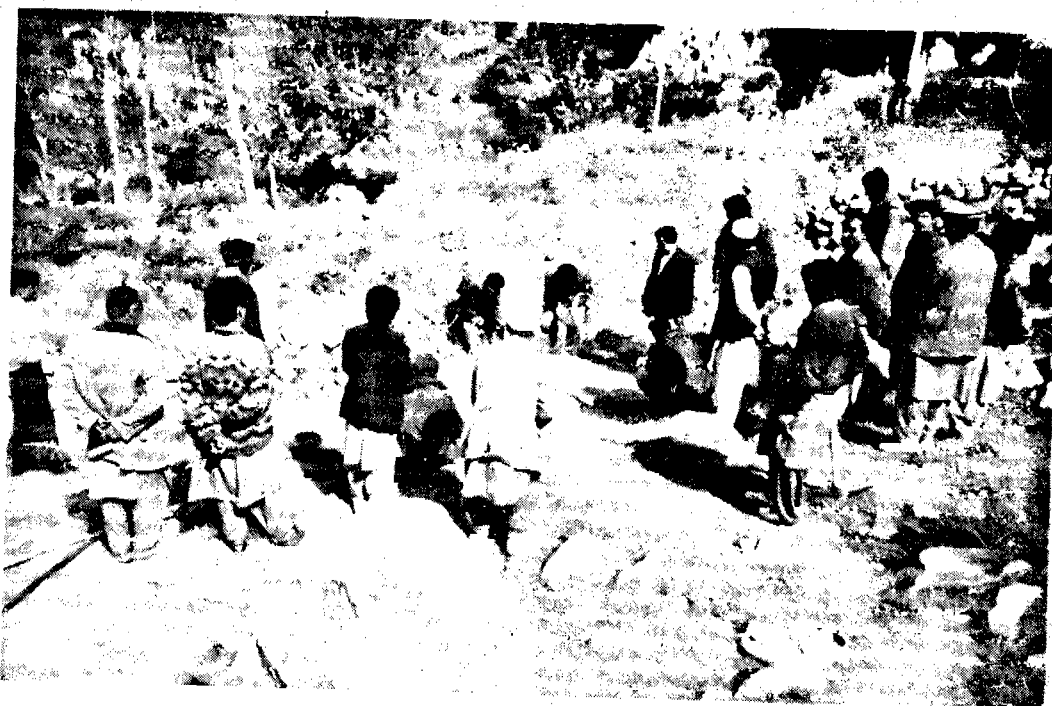
Figure 1. Villagers preparing site for storage reservoir in Ayeenabad, Gilgit.
