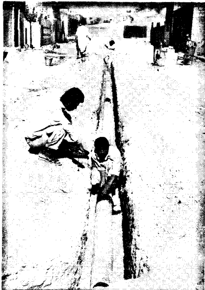
Lane activist supervises the construction of lane sewer in Ghaziabad
