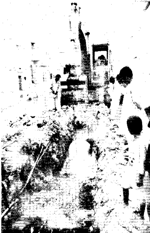
OPP-RTI member monitors the construction of main sewerage line in UC-3 Jamshed Town
