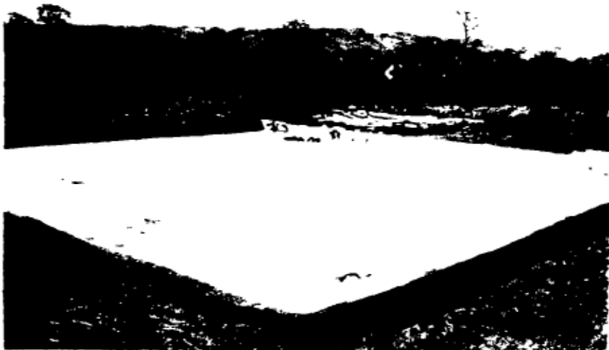
Plate 7.2 ...Mud/Dung Traditional Threshing Floor being used as a Catchment Apron for the same Tank near Shoshong.
