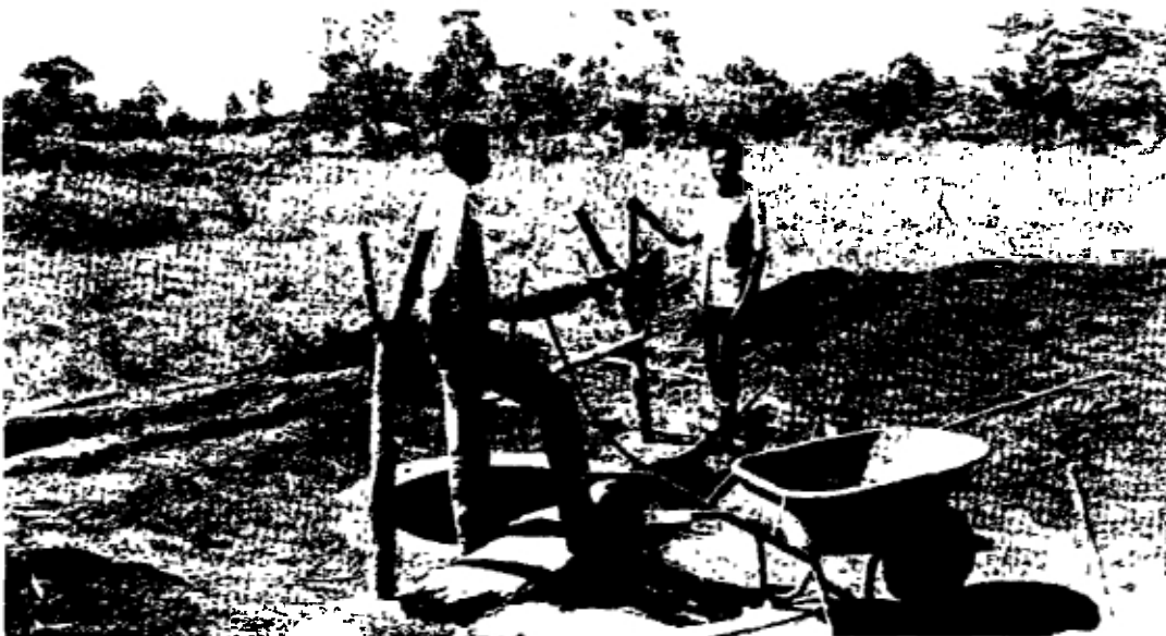
Construction of a hand dug well
