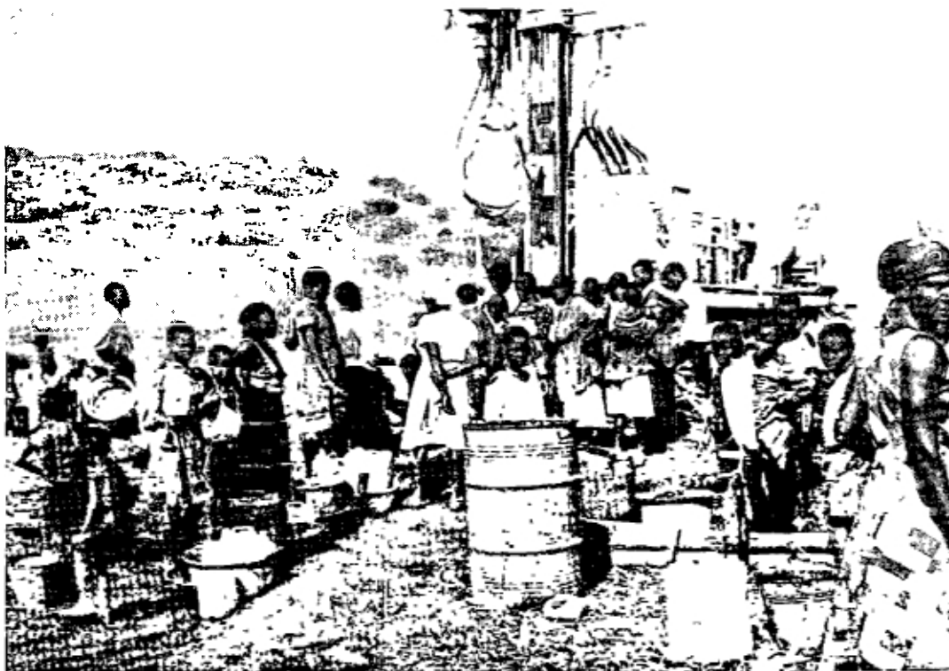
Drilling of a deep well
