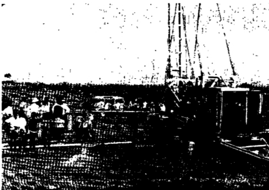
Borehole drilling
