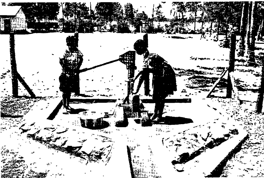
Borehole with hand pump; a ground water source
