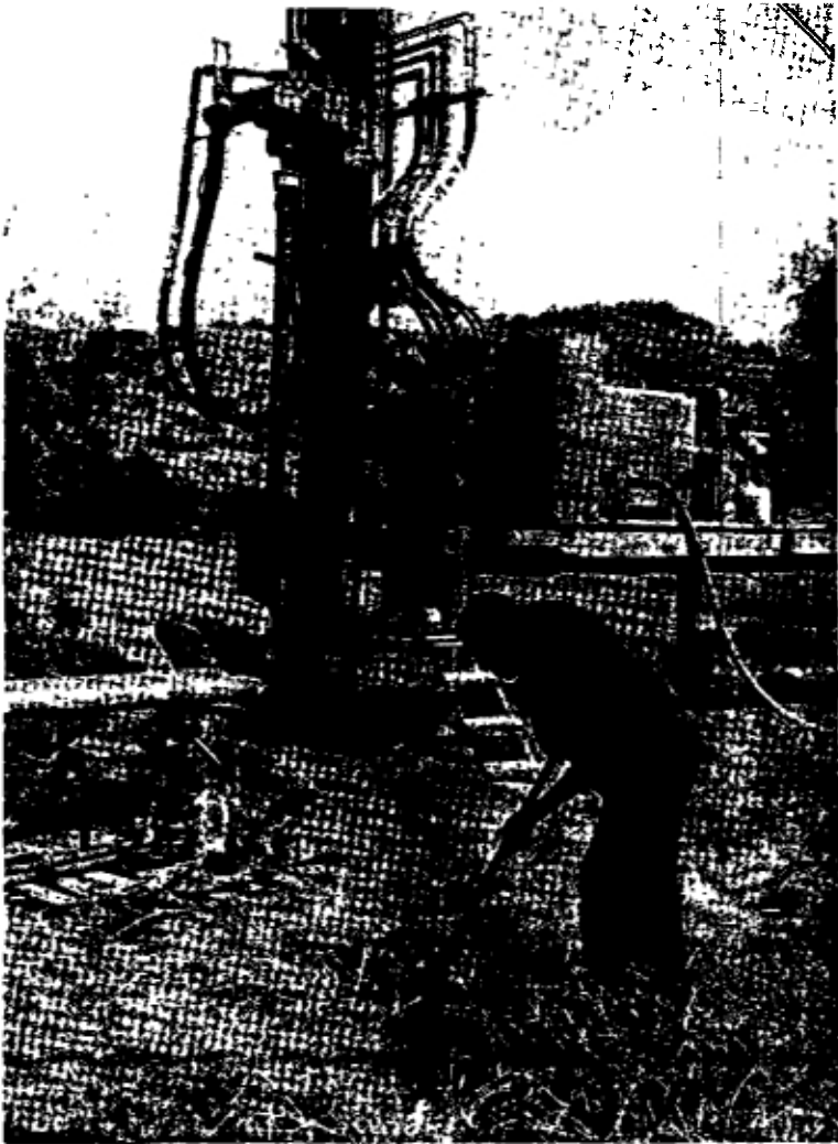
Borehole drilling
