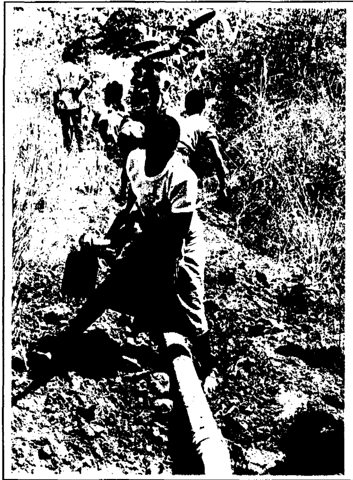
Digging of pipeline
