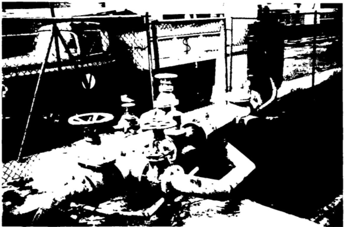
Figure 4.2 Production Meter Installation - Borehole No 15
