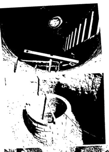
Since the diameter of the well was not circular, three pillars were added to provide additional support.
