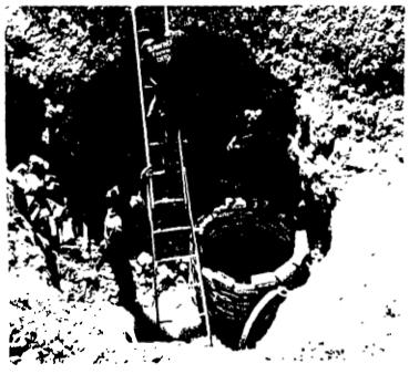
The construction has started with the porous concrete of ratio 1:1:4 (cement:sand:gravel) which is the foundation. The water could enter the well without hinderance. As construction goes on, backfilling is needed to an able the contractors to carry on with the lining work.
