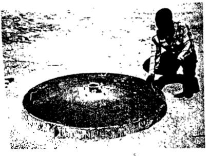
Making of the cover slab of a pump. The concrete is poured in the mould half full, then the reinforced bars are placed on top. Later the mould is filled with concrete. The bolts have to reach the reinforcement bars in order to keep the base plate in
