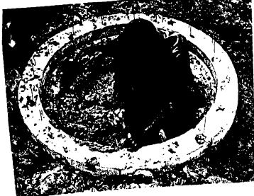
Reinforcement is then placed into the excavation made for the cutting ring, thereafter the mortar is poured inn. From there, lining continues. Also at every fourth course, a step and a reinforcement wire is placed. Since this method is sinking, people must dig inside in order to sink the well. Community is trained to do the work.
