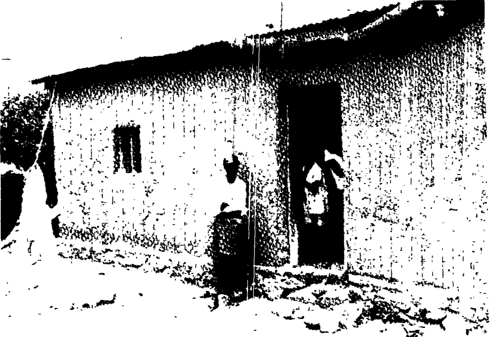
Plate 1. Roof Catchment with short gutter and a plastic bucket.
