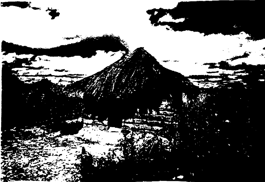
A latrine constructed with local materials.
