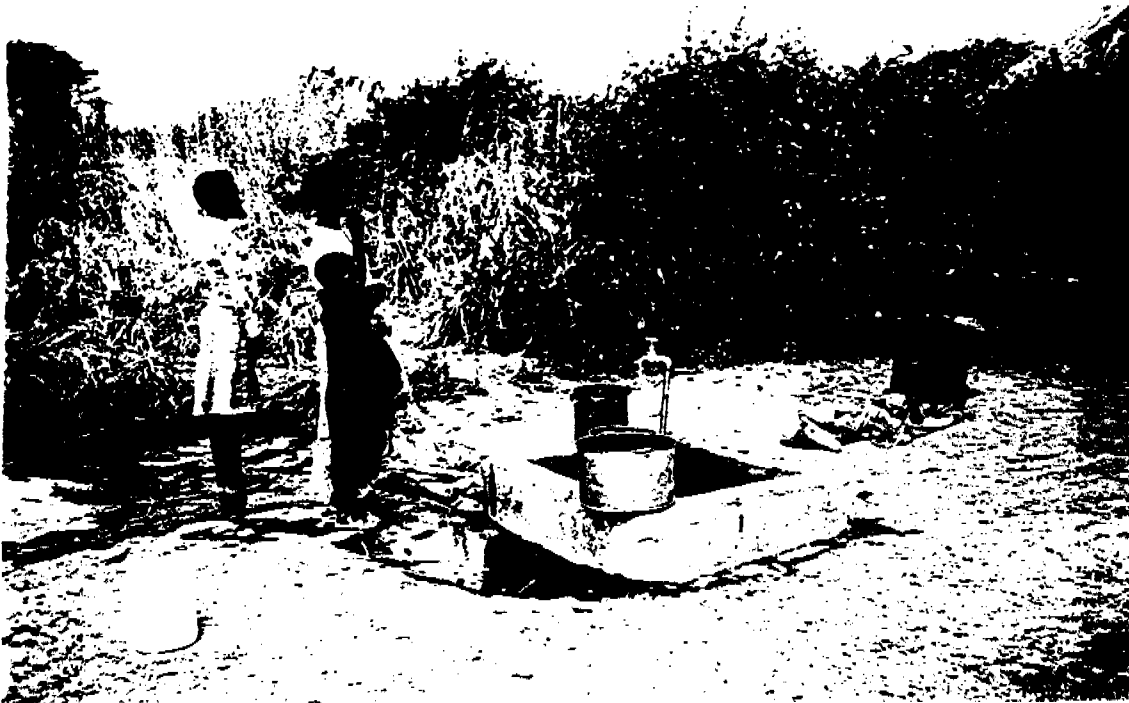
10. Chongwe: PSWS standpost. The drainage has to be improved.
