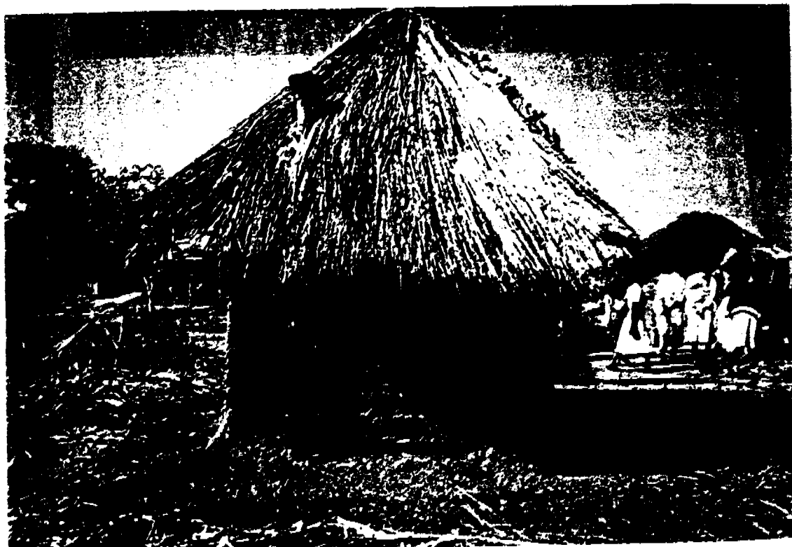
11. Mulimba: an improved pit latrine, built with local materials after a model developed through the PSWS project.
