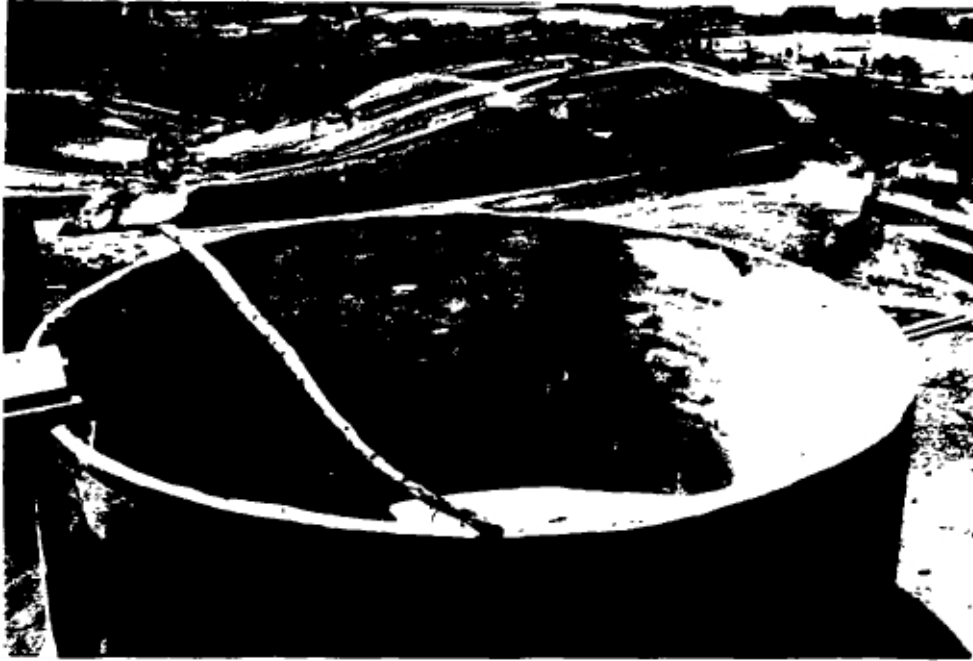
Photo 7. Experimental ferrocement water storage tank.
