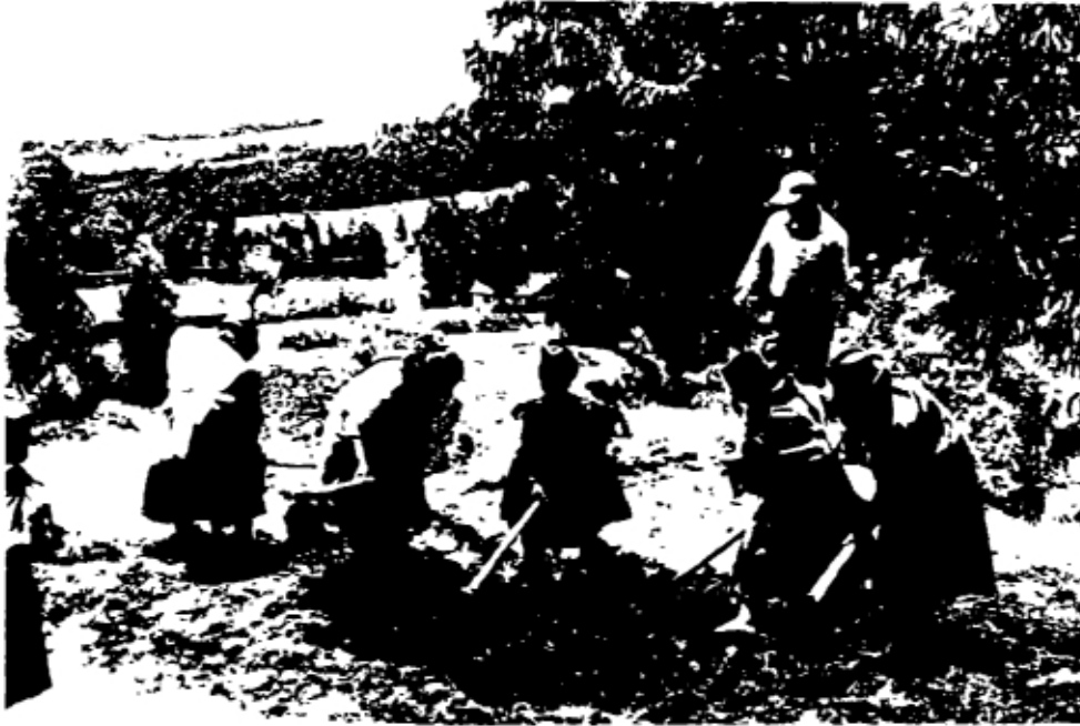
Photo 1. Women from rural community working on trenches for water pipe.
