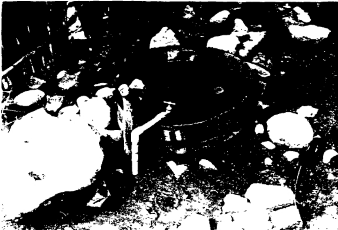
Photo 1. Water tap installed close to ground level due to low pressure - La Criba.
