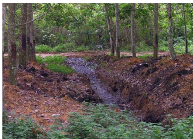
In using plantation sites for trenching, IWK can reduce its land costs and contribute to the productive reuse of septage. Trenching might only be appropriate for less urban areas; it also requires longer hauls, and consistent monitoring for groundwater contamination.
