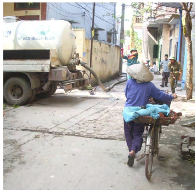
A desludging services operator empties a neighborhood septic tank. The accessibility of septic tanks can pose a significant challenge for septage collectors, and serve as a deterrent to more frequent desludging.
