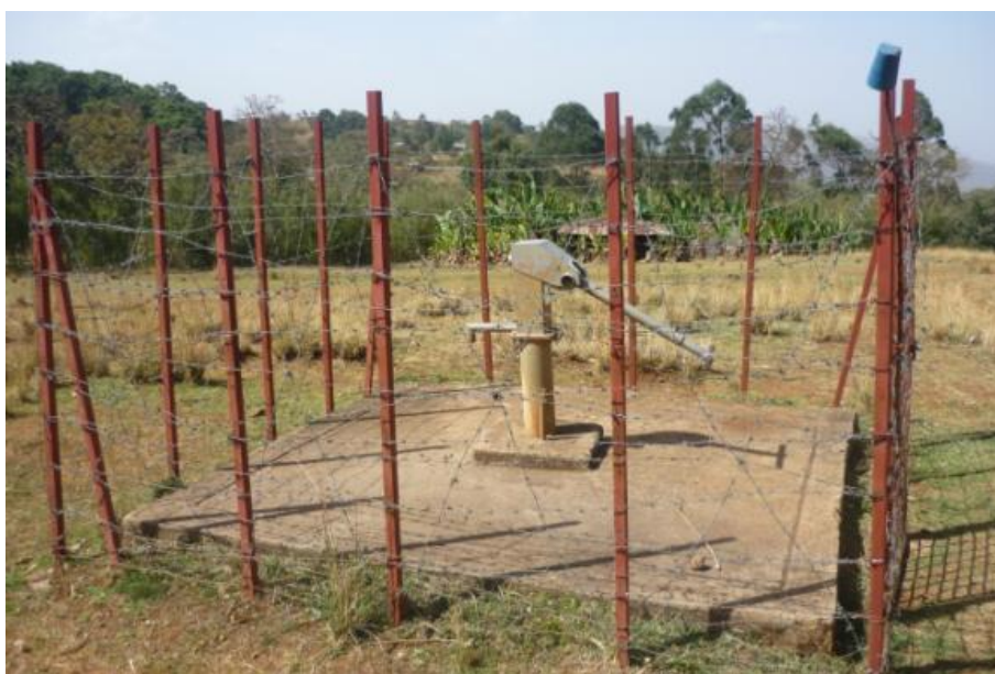
Figure 4.9: The non-functional MSW fitted with a hand pump
