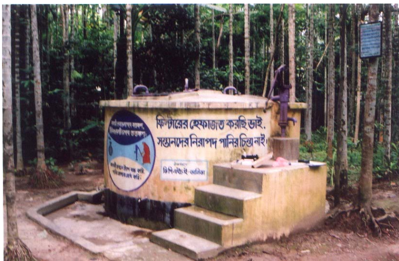
Figure 2.8: A pond sand filter
