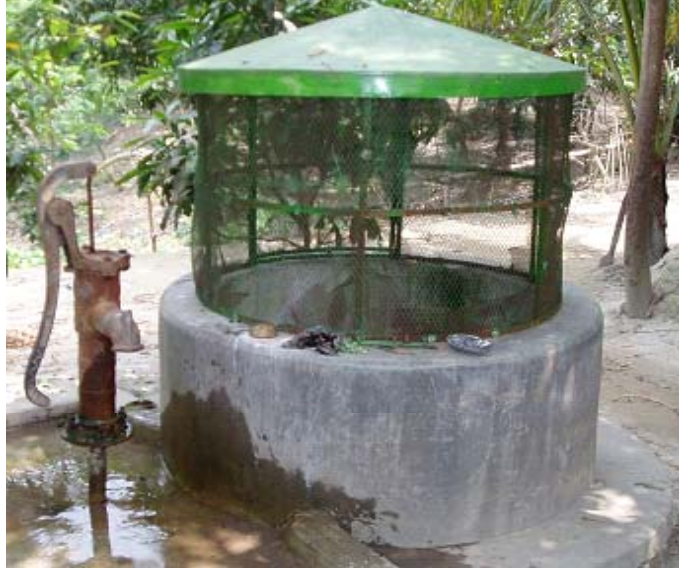
Figure 2.4: Improved dug well with opening for entry of light and air
