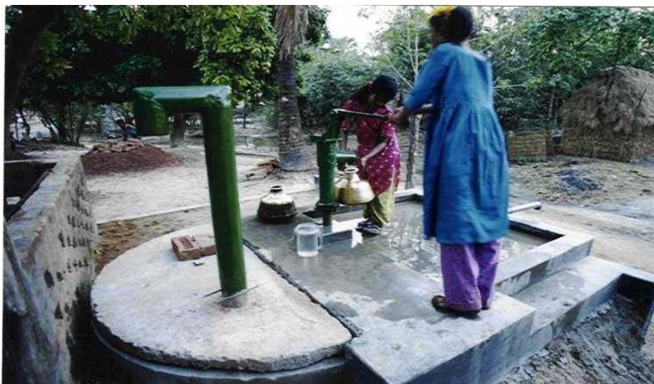
Figure 2.3: Water collection from a closed dug/ring well by handpump
