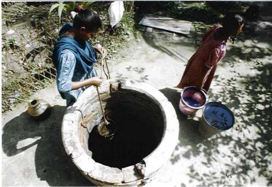
Figure 2.2: Water collection from an open dug well
